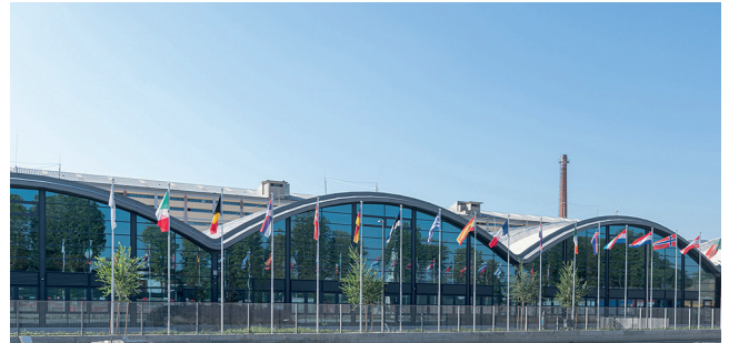
FIGURE 1 The new data centre in Bologna.
