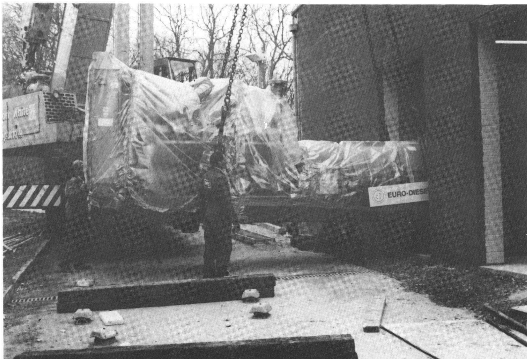
Heavy equipment being lifted into the new energy centre
