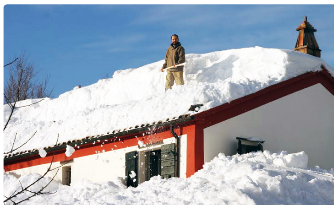
Figure 6 A colleague rushing to clear packed snow because of fear the roof would collapse under the weight of incoming new snow (taken on the 7 February before the second big snowfall).
