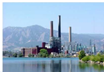
Valmont Power Plant ~200 MegaWatts Boulder, CO
